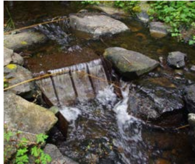
Photograph 2: Screened inlet pipe in Millard Creek main stem, showing waterflow – 22 nd of August 2012
